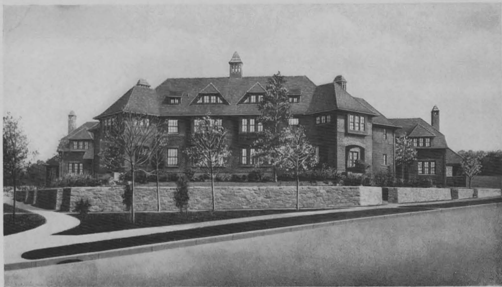
A GROUP OF FOUR HOUSES AT THE INTERSECTION OF GREENWAY NORTH AND MARKWOOD ROAD
