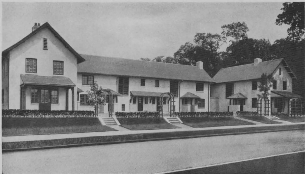
A GROUP OF FOUR HOUSES ON GREENWAY NORTH
