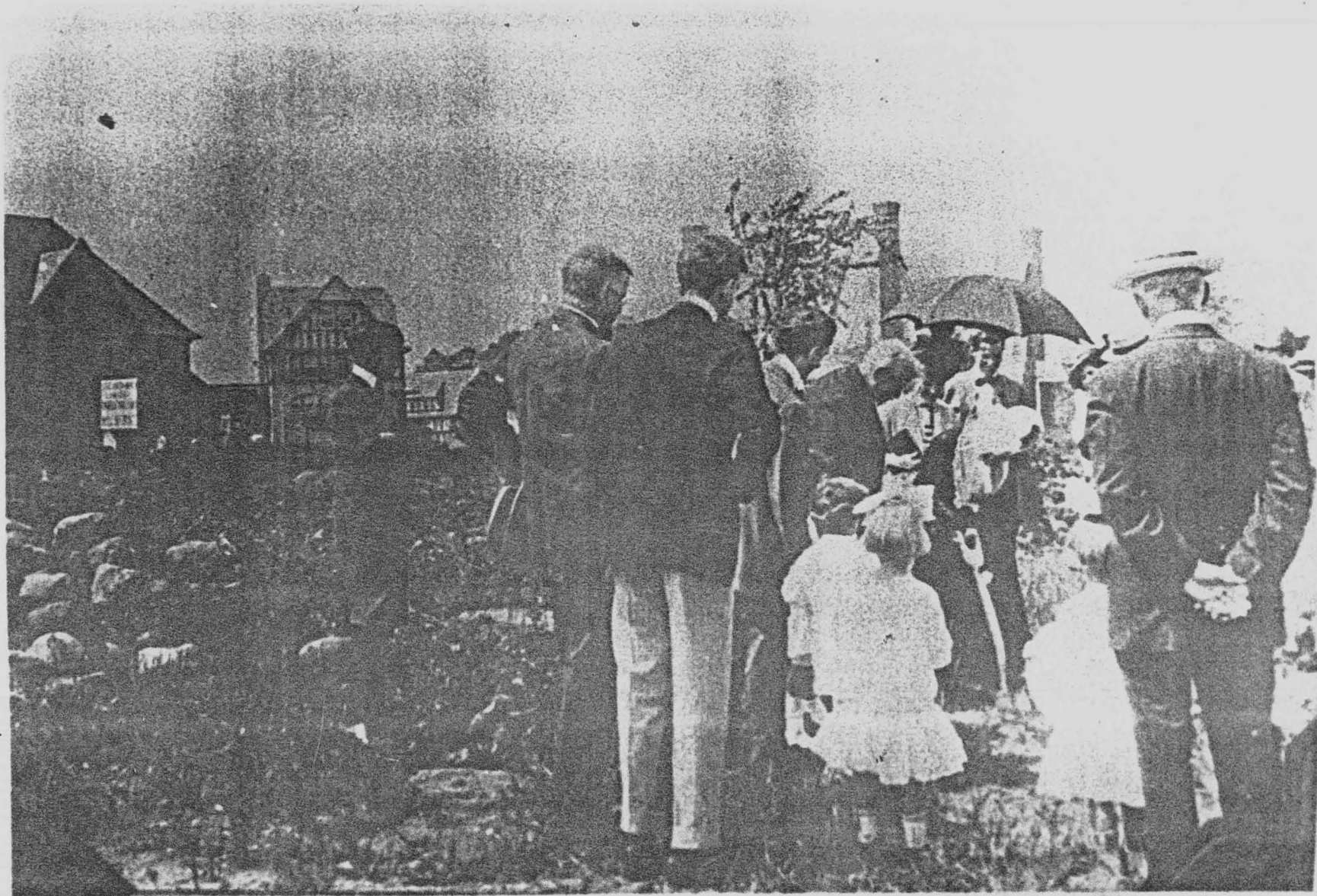
Ground breaking: Church in the Gardens 1914
