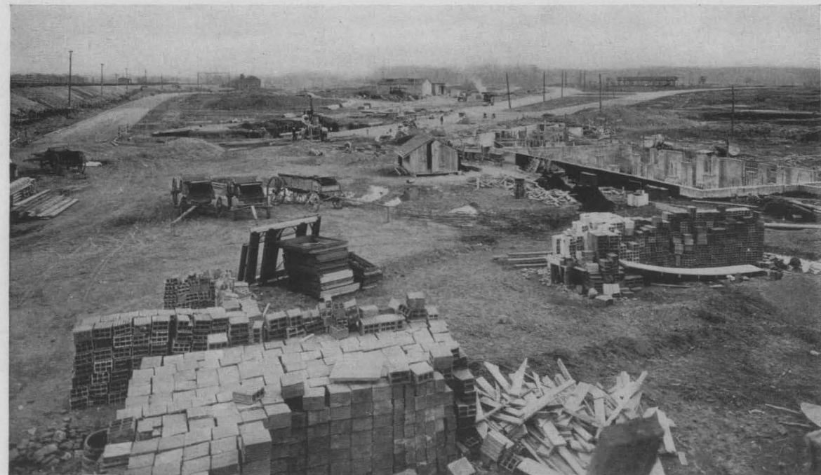
BUILDING OPERATIONS, FOREST HILLS INN, NOVEMBER 1910
