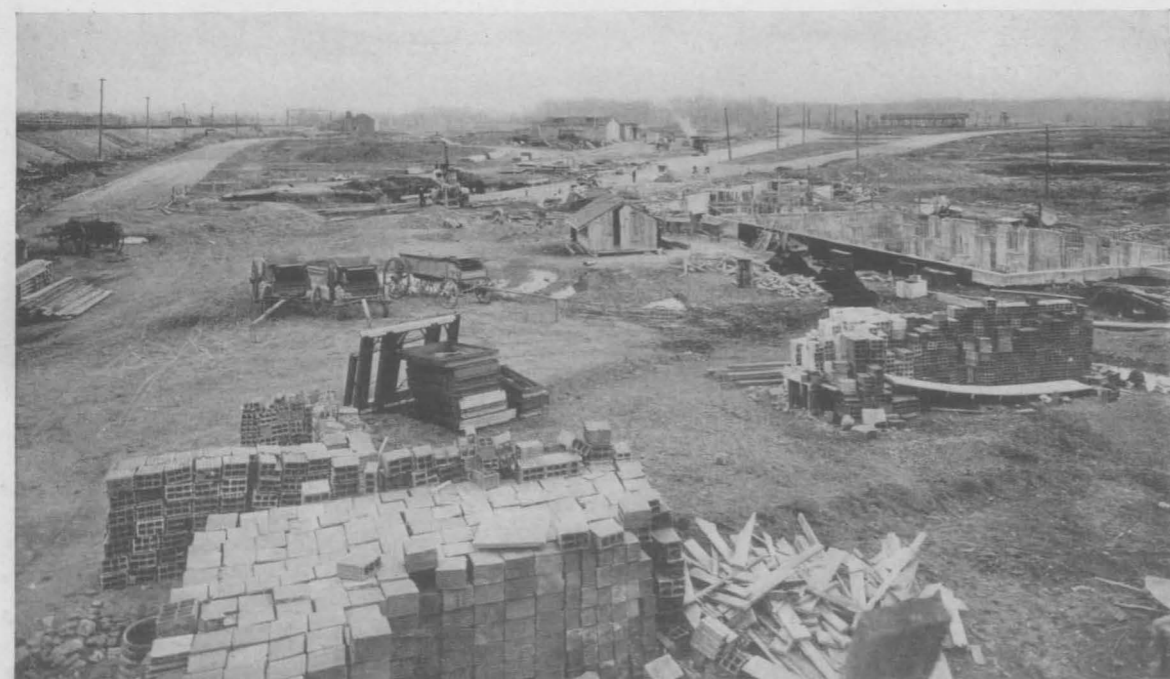
BUILDING OPERATIONS, FOREST HILLS INN, NOVEMBER 1910
