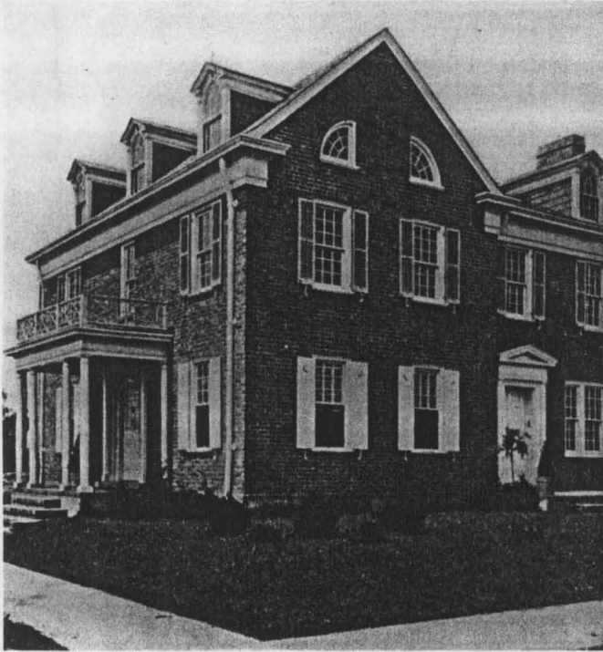
Group house, Willet Avenue to Middletown Street between Shelton and Colonial Avenues, Jamaica, Queens. Electus D. Litchfield, 1914. A 1914 view of a typical end unit in a group of four houses. CU
