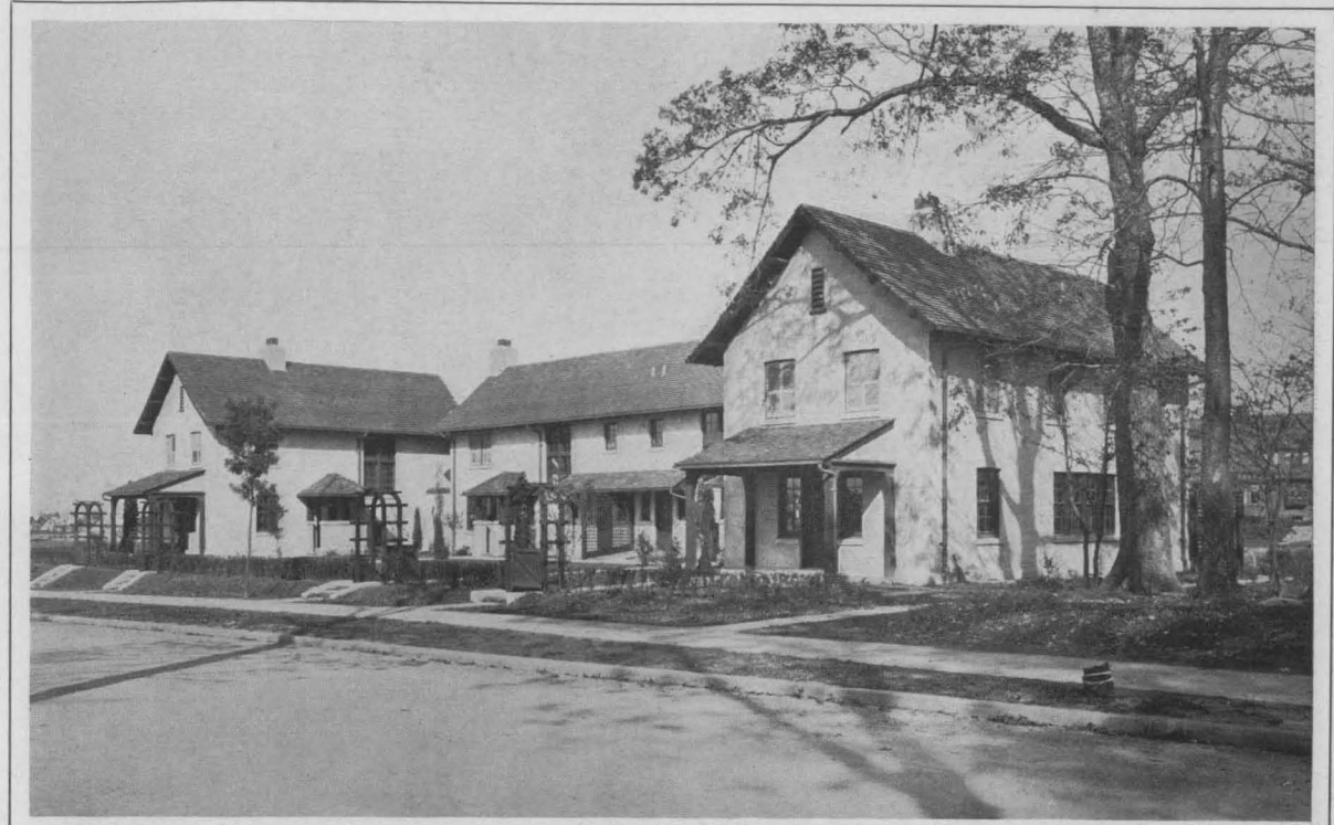
GROUP XIII LOOKING NORTH
