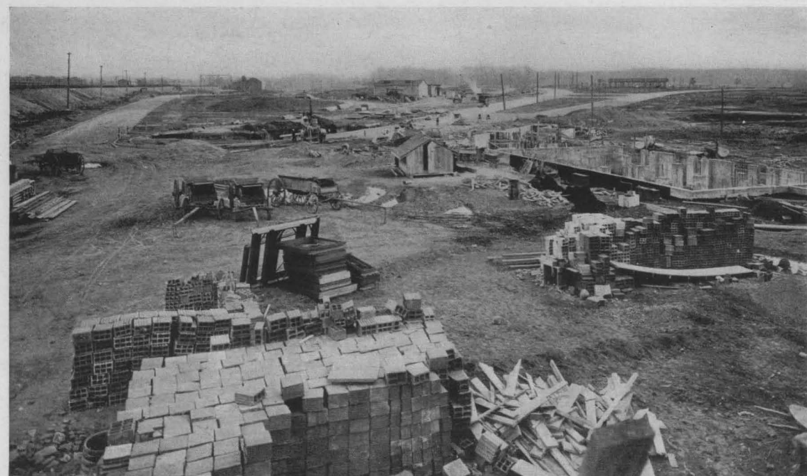
BUILDING OPERATIONS, FOREST HILLS INN, NOVEMBER 1910
