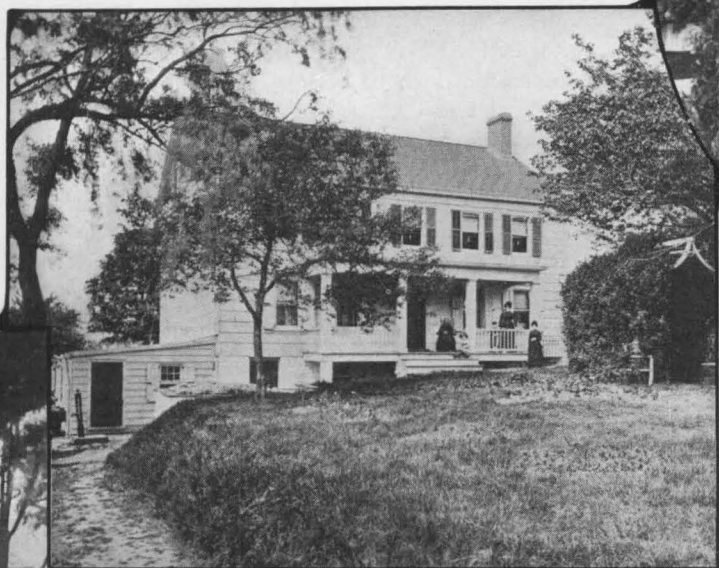
McCown-Backus House (above). Stood on Queens Boulevard until ten years ago, when torn down. It was 160 years old, one of the best of Whitepot houses.
