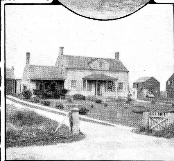
The Judge Jonathan T. Furman House (above), standing on Dry Harbor Road, built in 1750, and is in excellent condition.
