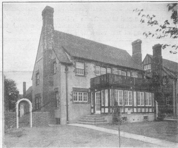
SIX-ROOM SEMI-DETACHED HOUSE ON WHITSON STREET—JUST COMPLETED BY THE FOREST HILLS GARDENS HOMES CO.
